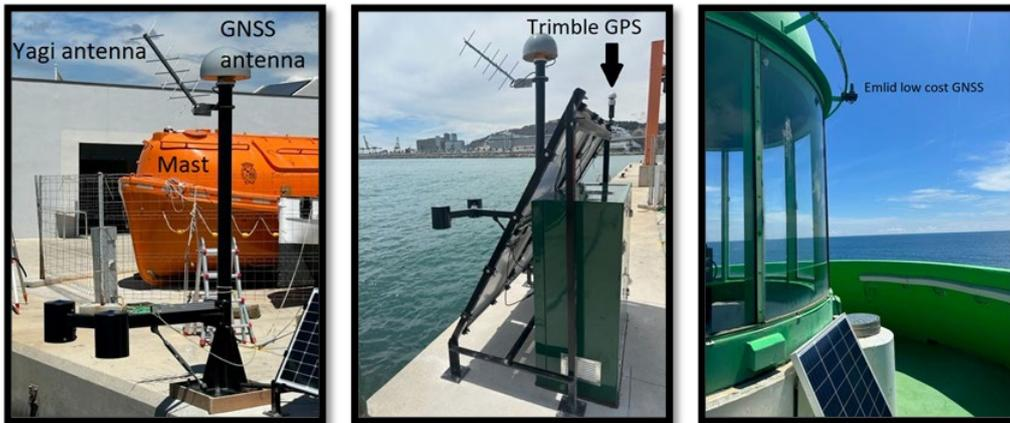
Figure 8. Completed tide gauge installation at Barcelona primary site (left) and (middle) and secondary site (right)
