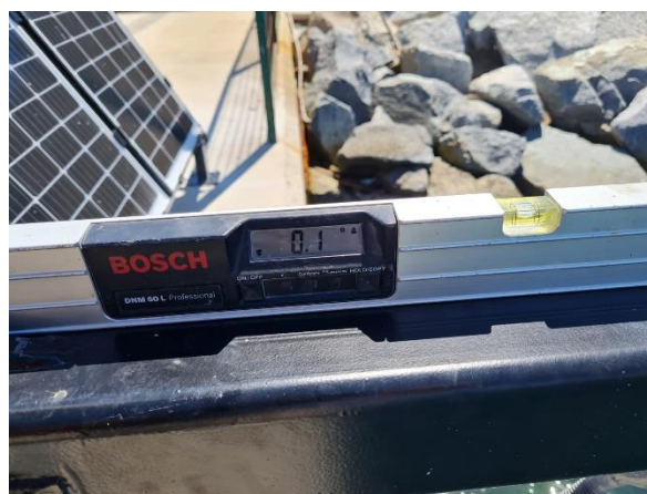
Figure 18 Levelling the radar arm.
