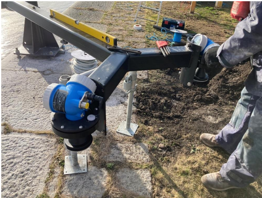
Figure 17 Installing the radar sensors.
