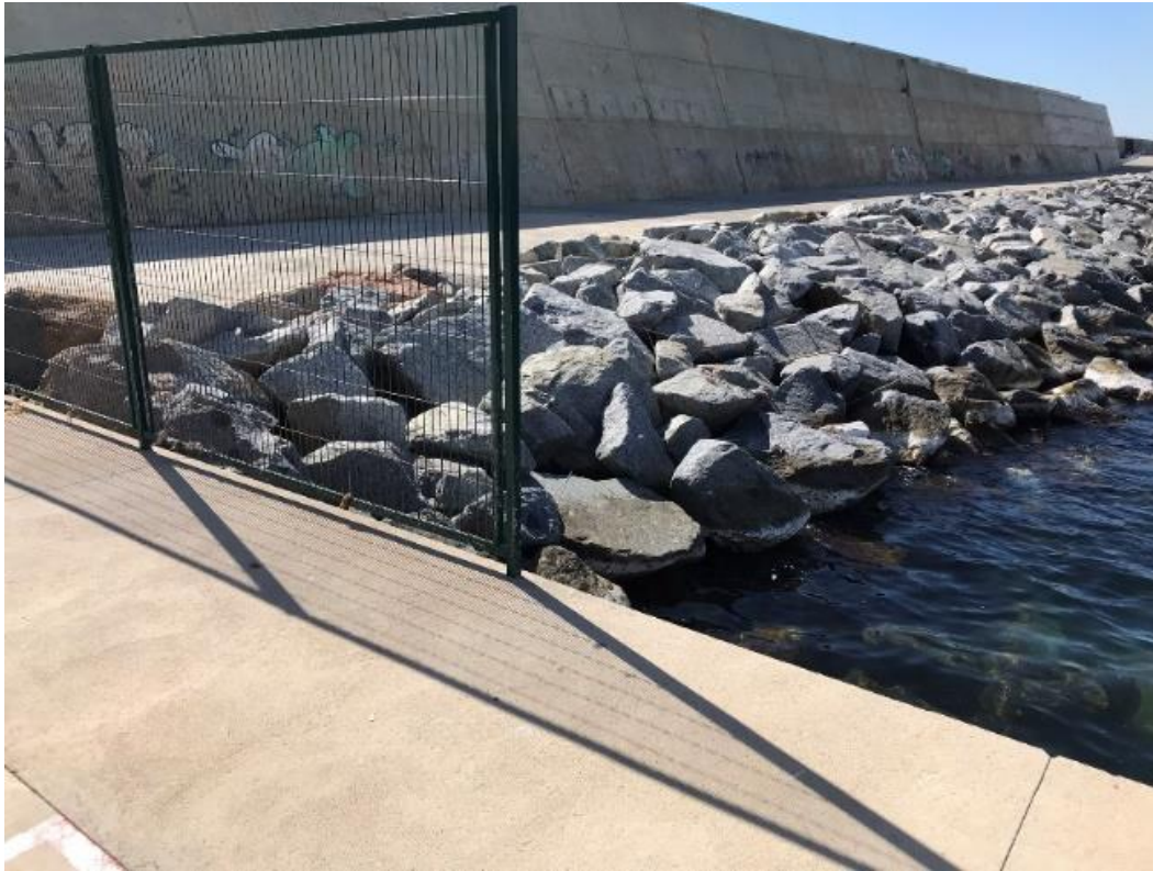
Figure 3 Location of solar panels
