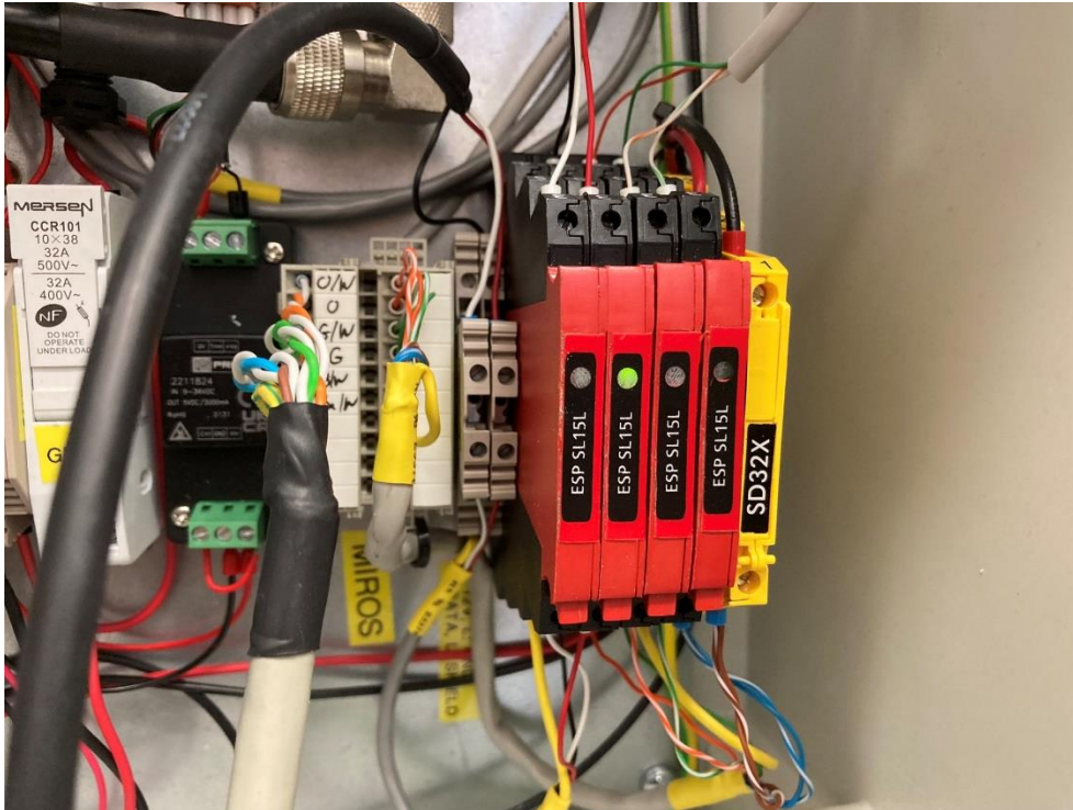
Figure 21 Radar sensor connections.
