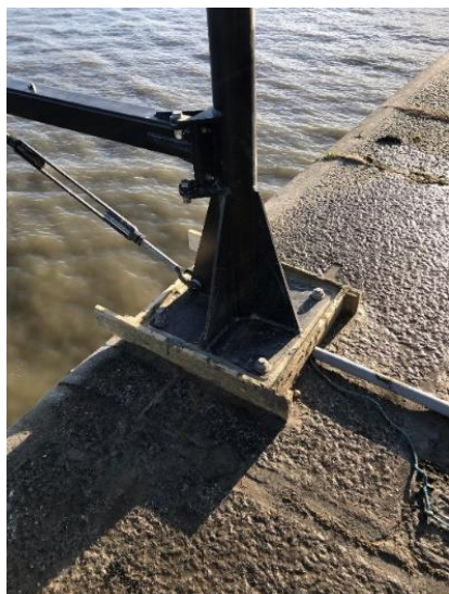
Figure 54 Mould filled with cementitious grout.
