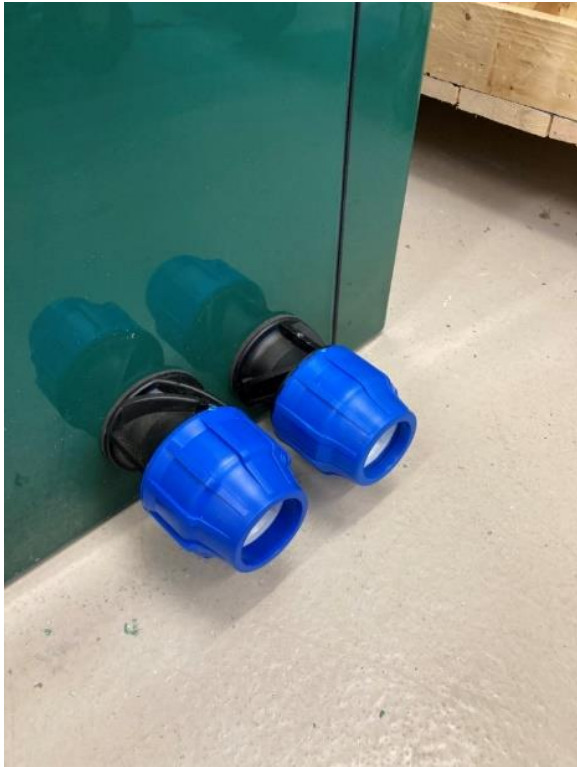
Figure 12 Cable glands for conduit. Location of the entry holes are to be determined during installation.
