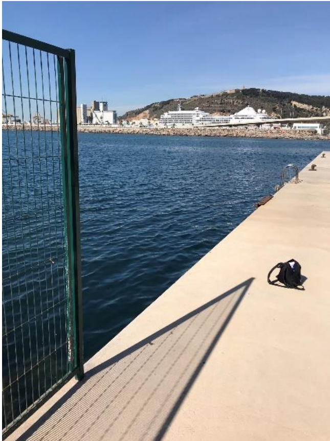
Figure 4 Quayside for installation
