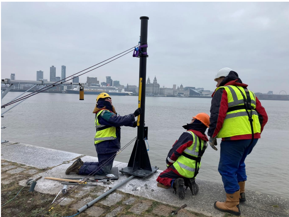
Figure 11 Levelling the GNSS mast.
