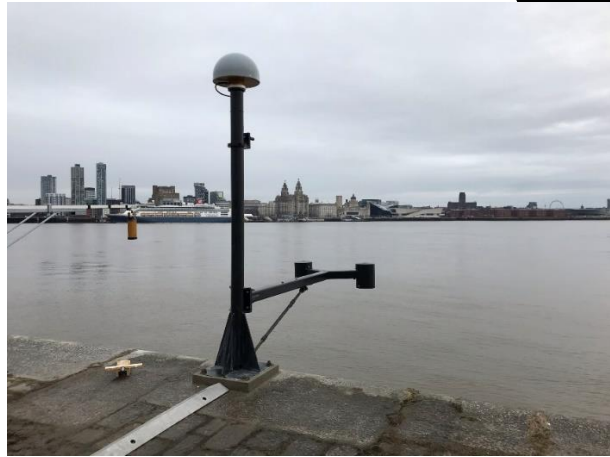
Figure 37 Finished installation with grout base.
