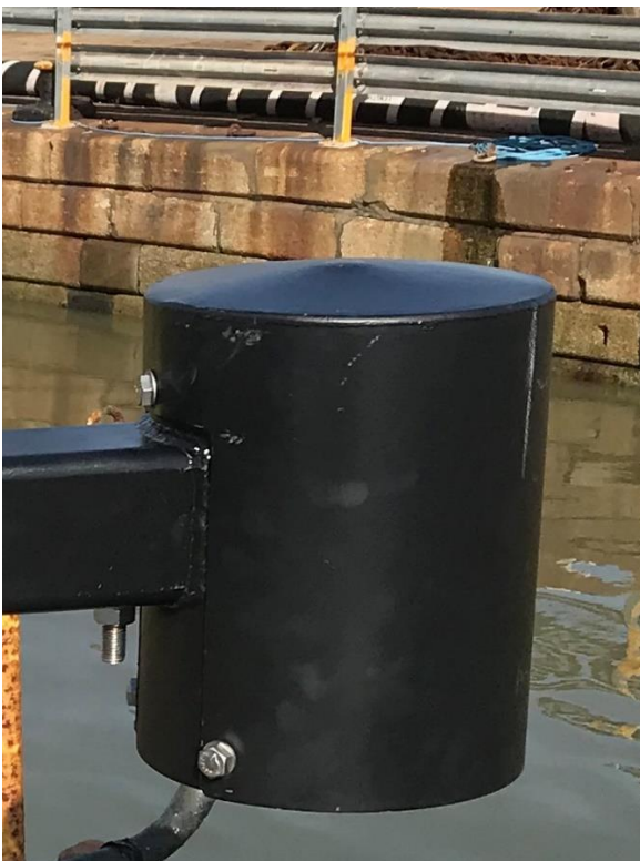
Figure 35 Radar protective cover.
