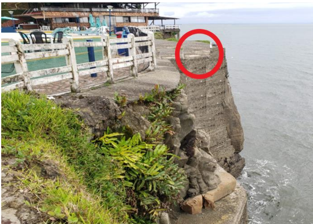
Figure 4 GNSS mast installation site circled in red.
