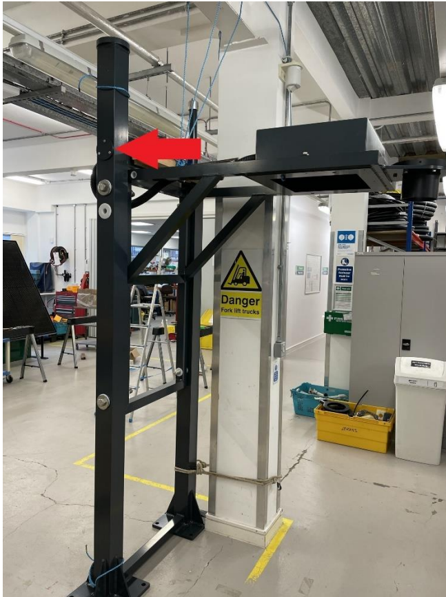
Figure 16 Cable access cover in A frame.
