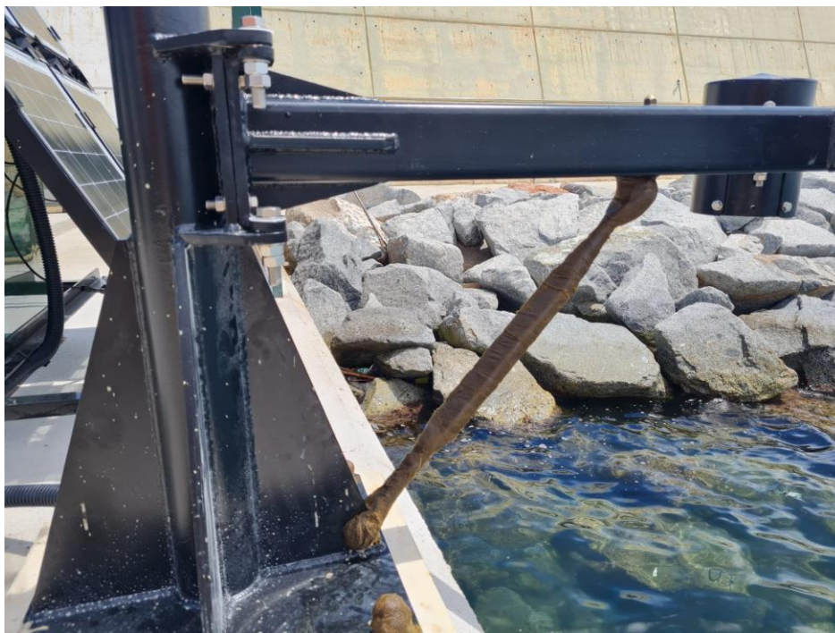
Figure 53 Denzo tape applied to turnbuckle and bolts.
