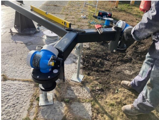
Figure 23 Installing the radar sensors.
