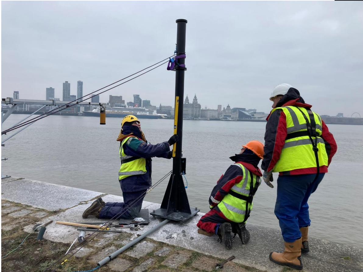
Figure 14 Levelling the GNSS mast with conduit in place.
