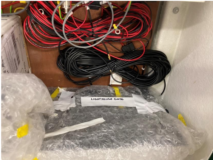
Figure 47 Low cost GNSS items.
