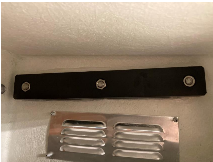
Figure 14 Solar panel frame support piece.
