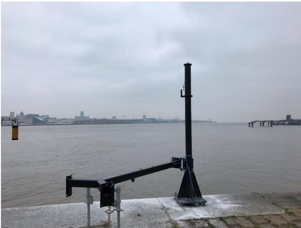
Figure 6 Radar arm swung inwards at Alfred Dock, Birkenhead, UK.
