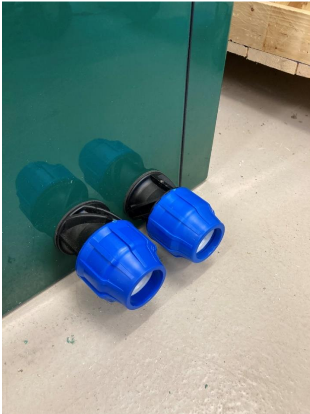
Figure 15 Cable glands for conduit.
