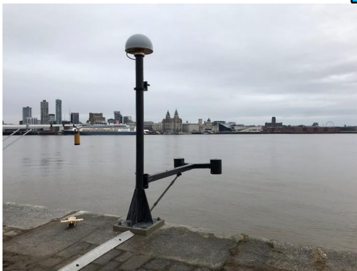
Figure 55 Finished installation with grout base.
